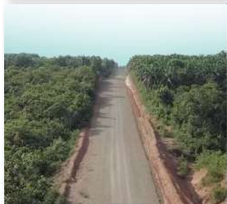
Dedicated coal hauling road
