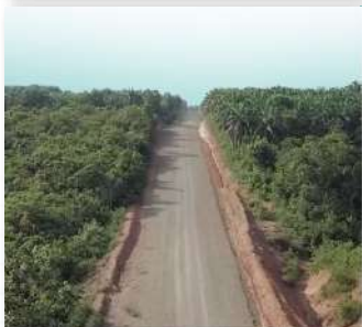
Dedicated coal hauling road
