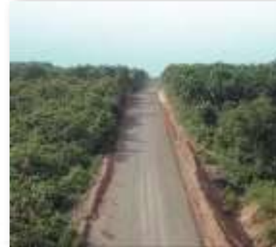
Dedicated coal hauling road
