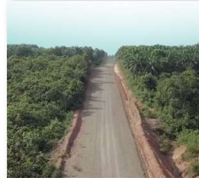
Dedicated coal hauling road
