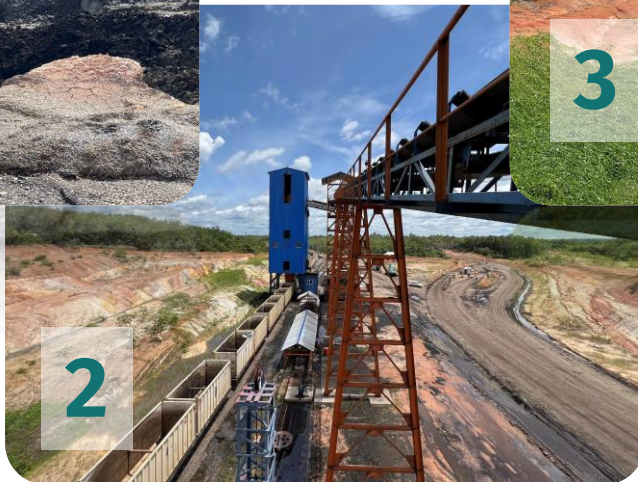
Gunung Megang Loading Station with Train Loading System (TLS)
